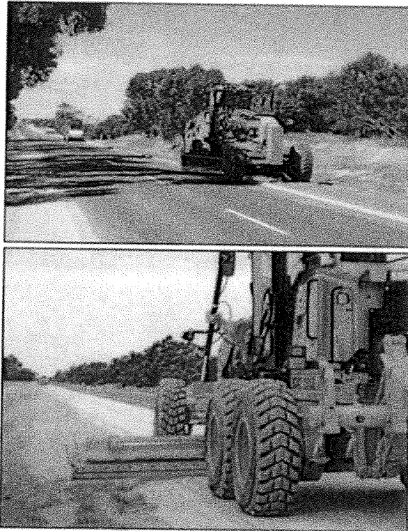
PDE final trimming with grader
